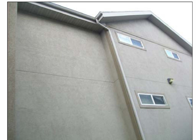
RISER TO ATTIC
