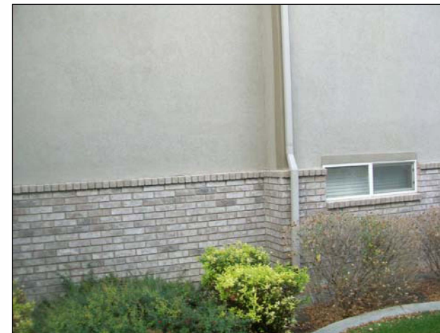
TYP. NOP WITH RAIN GUTTER AND MD RISER TO ATTIC
